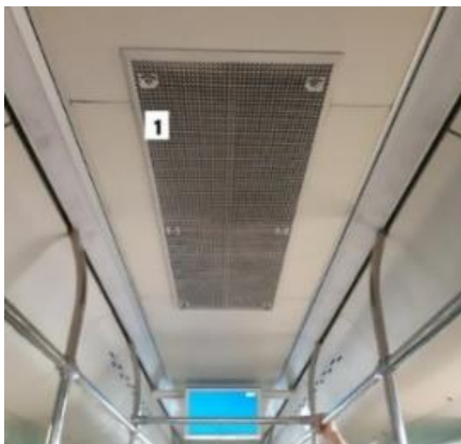
Figure 9 The air filter of the air conditioning system in the ceiling of the bus: 1 the air filter in the metallic frame, viewed from the bus interior. (Daniela Obitková 2023)
